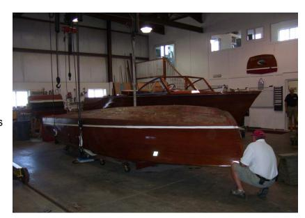
tops of our new stringers. We spent a little time shimming so we knew the boat was set level (just so we could double check measurements and make sure we were keeping the shape of the boat correct while working on the bottom) and then we were ready to rip off that old planking.
